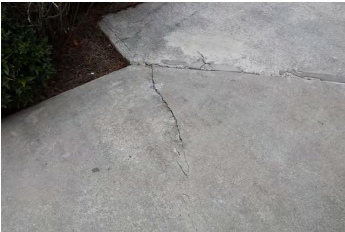
Clean out cracks and fill with self-leveling concrete sealer
