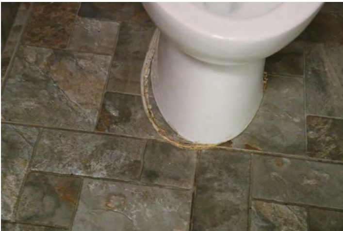
Reposition toilet and recaulk
