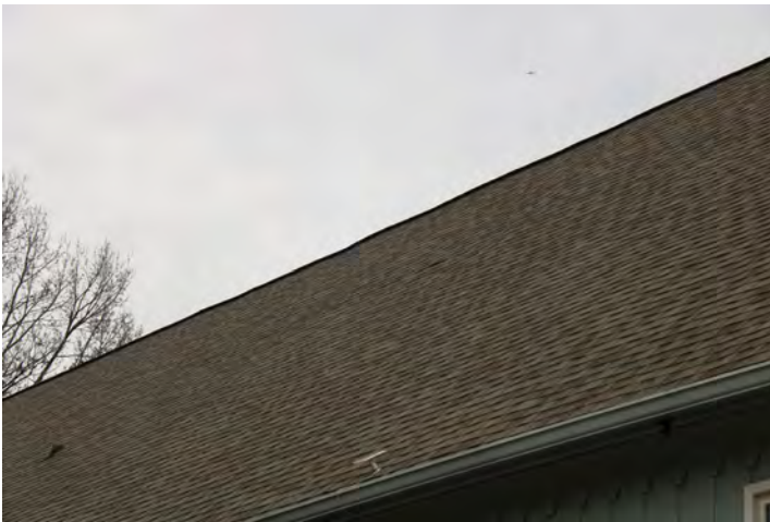
Parish Hall roofing showed no deficiencies
