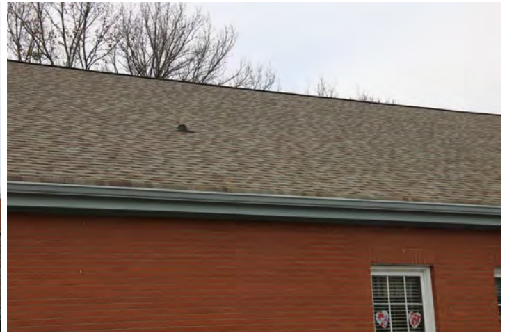
Dimensional shingle on Education Building is in good condition
