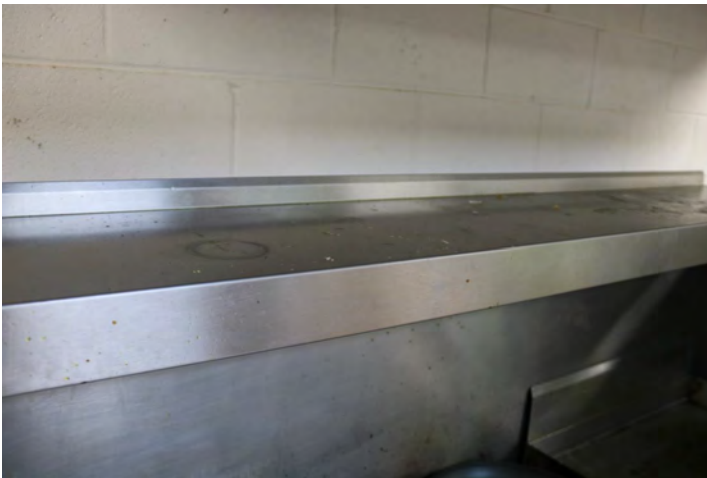
Clean dust and grease from shelf above stove
