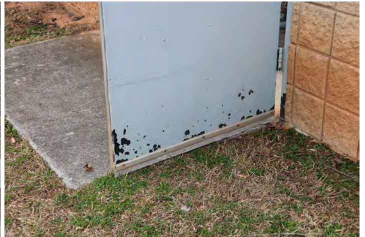
Sand damaged area and repaint door
