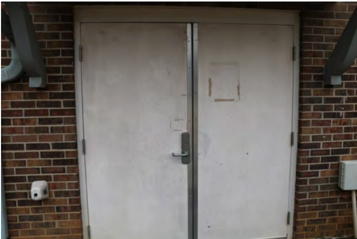
Clean doors and repaint as necessary
