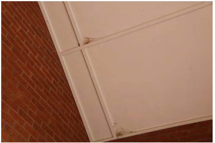
Clean webs from ceiling areas
