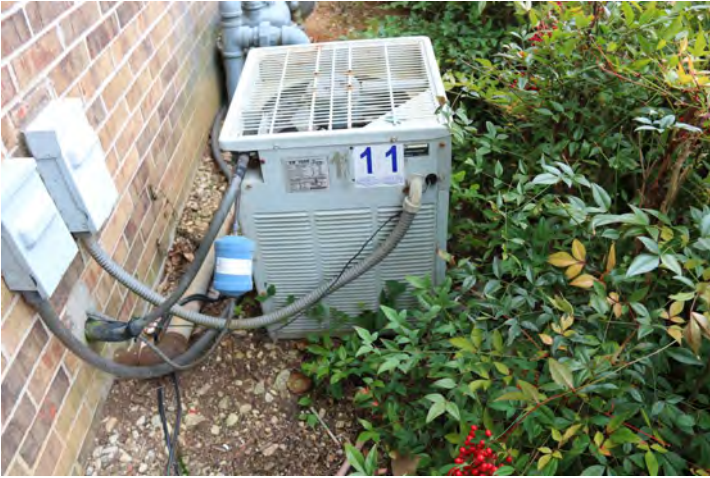
The area around HVAC units is free from vegetation
