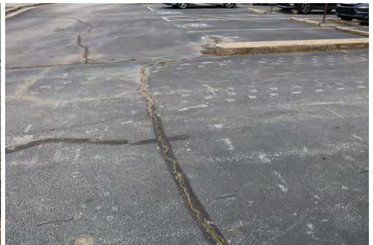
Remove vegetation from cracks and fill with sealer
