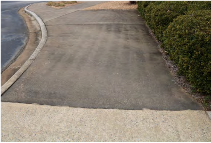
Pressure wash sidewalks to remove soil accumulation
