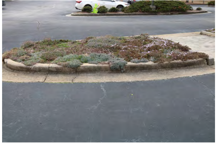
Trim vegetation along curb edge
