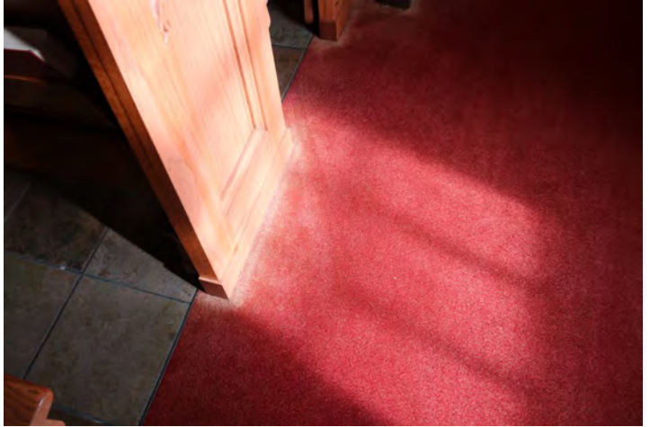
Accumulated soil appears as discoloration
