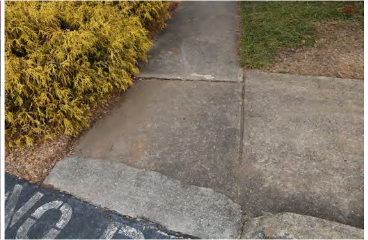
Grind down uneven transitions
