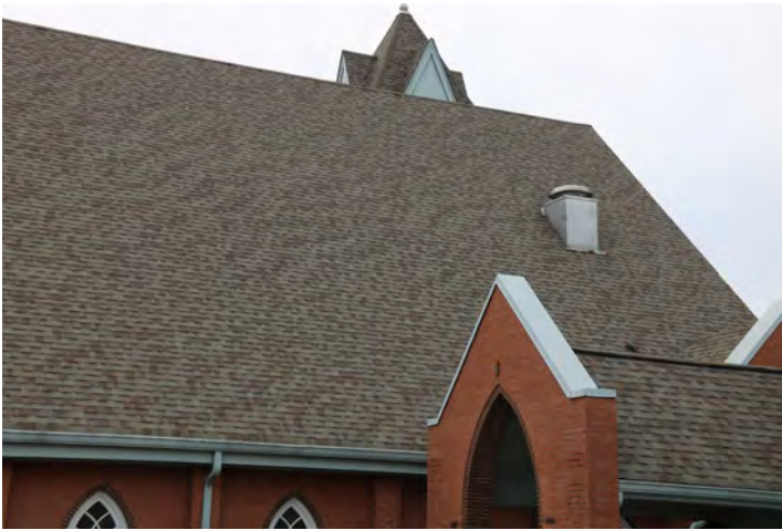
The church and office roofing is in good condition
