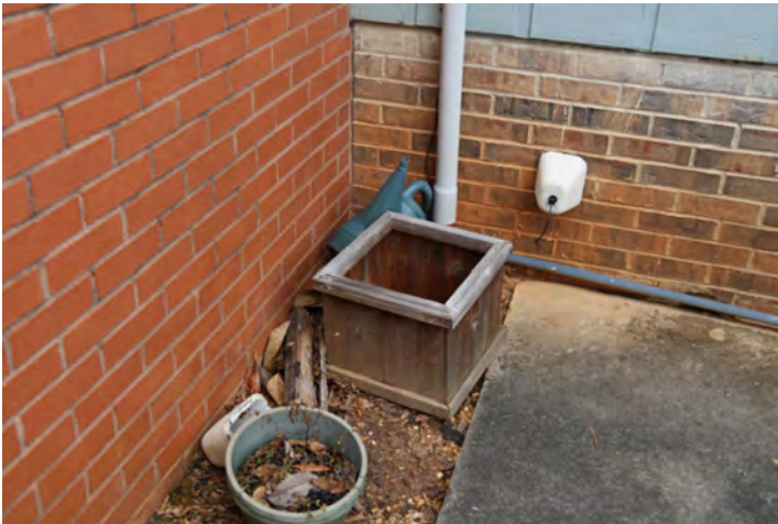
Remove debris and equipment from along building walls
