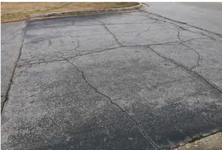
Clean cracks and fill with sealer
