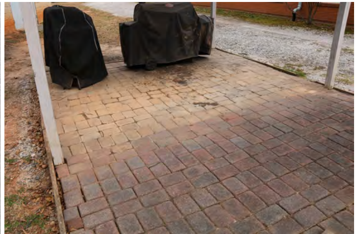
Pressure wash patio and fill joints with polymeric paver sand
