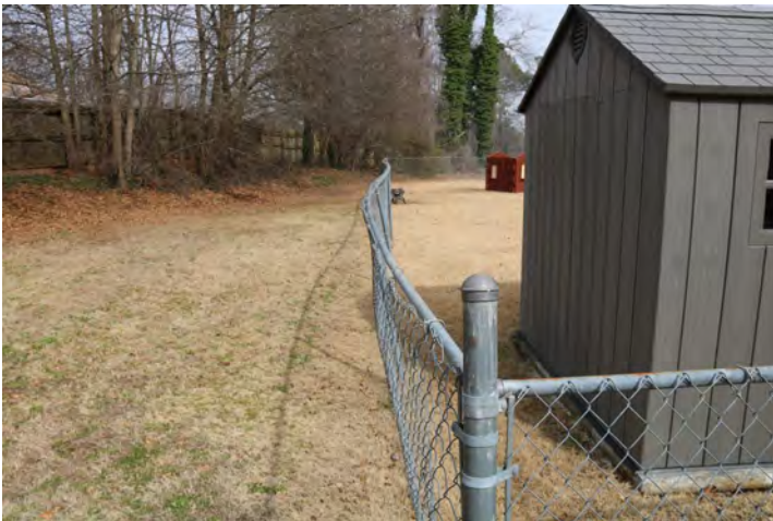
Fence posts appear loose
