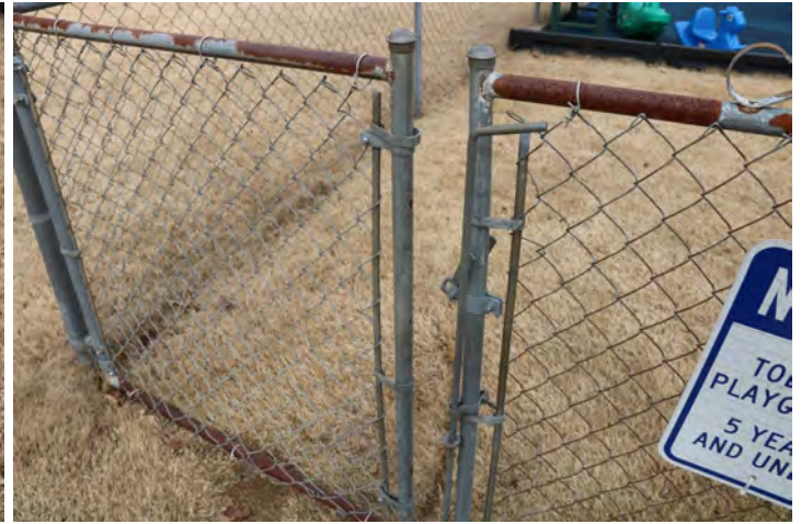
Rust on fence and gate rails
