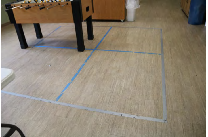
Remove worn tape and adhesive residue from flooring
